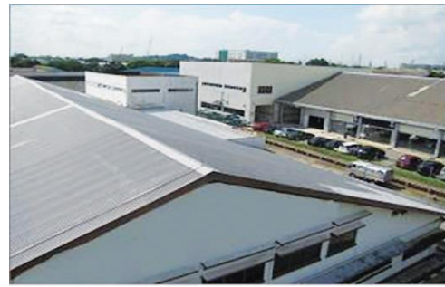
Metal roof of industrial
