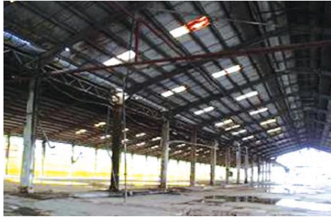
Industrial building with skylight
