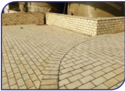
Acid & Alkali Proof Bricks Lining
