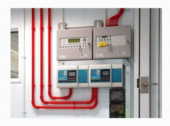
This can be the first level of fire security in premises where the air would be sampled continuously using suction pipes which pull the air into the aspiration detector. Even minimal amount of smoke would give a warning alarm, so that the premises can be checked. This can be installed in all critical areas.
