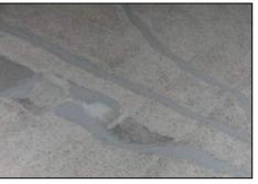
Weak concrete must be removed and surface defects such as blowholes and voids must be fully exposed. Cut all crack by concrete cutter & repair the substrate by Sikadur 31
