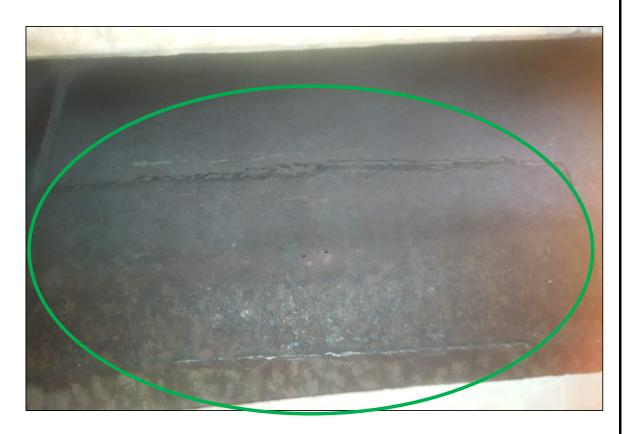
**Remark:** one metal sheet welded here and creat slope hence now no any material collect here.
